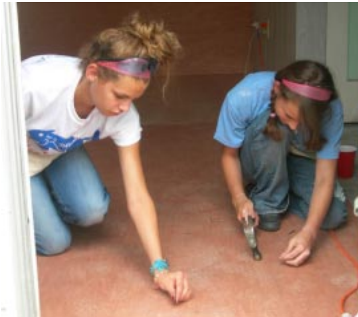
Ally and Alex, preparing the floor
